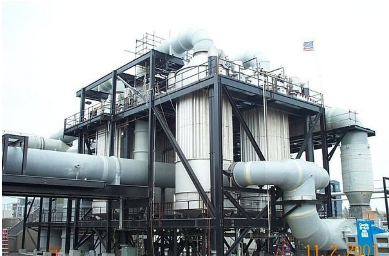
Figure 6 – SonicKleen WESP on B-218 Rotary Kiln
