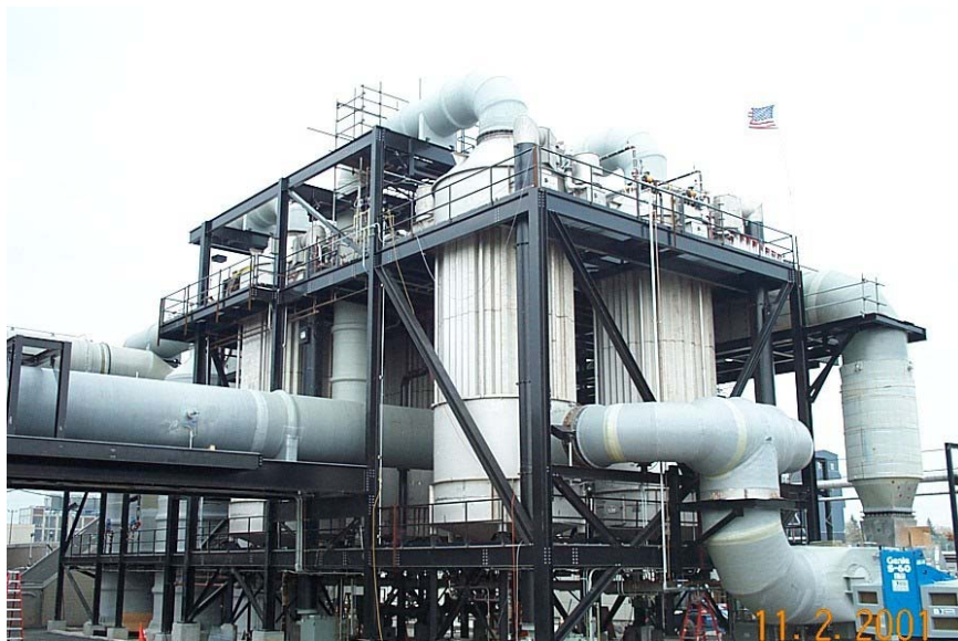
Figure 8. Typical TurboSonic WESP on a hazardous waste incinerator.
