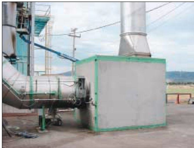
Extra set of mesh pads between wet ESP and RTO at LaGrande.
